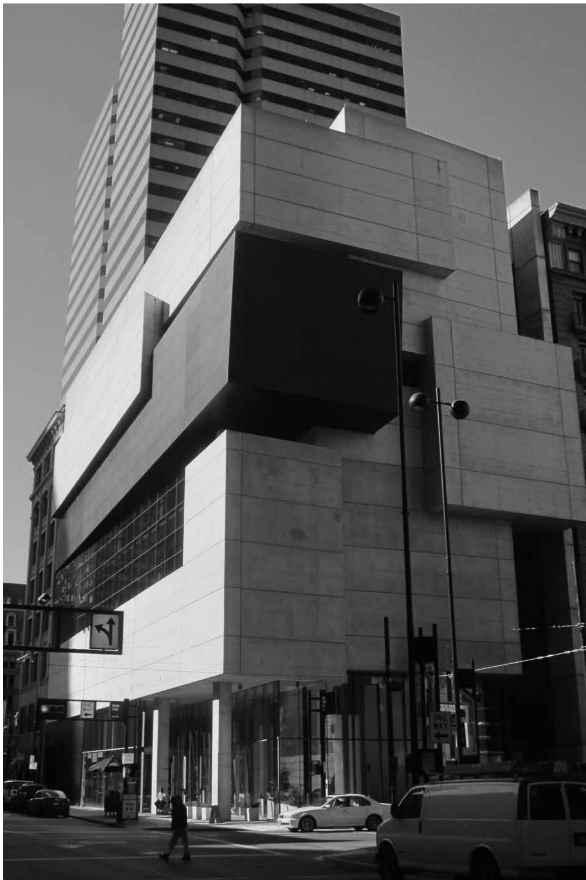
5 CAC, with Walnut Street facade in full view.
